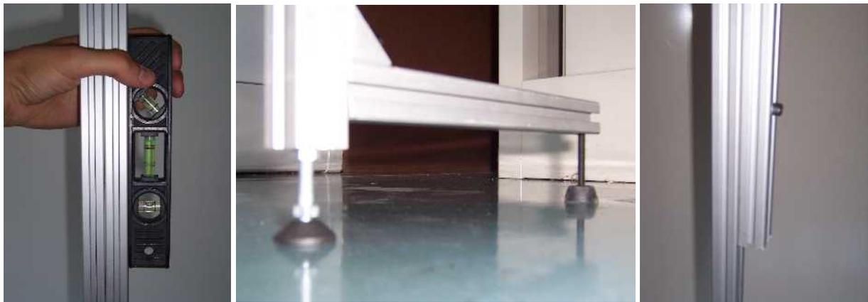
*Positioning a pole taking care to correct every possible skew with the spirit level.*
