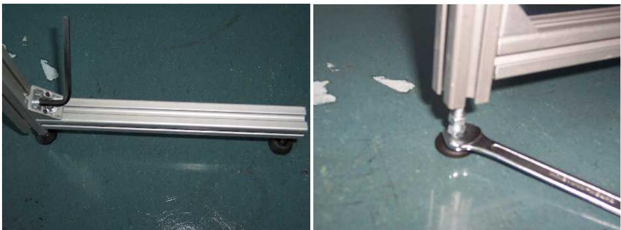
*Fixing a pole to the floor; both to avoid rotation (left) and translation (right).*
